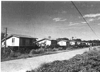
Fig. 300 Low cost housing estate in Rajang Town. (Photo: Lim Yu Seng)
