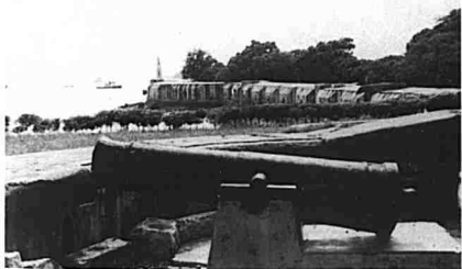
Fig. 117 The Cannon Platform built at Humen Town by Lin Zexu during the Opium War.
