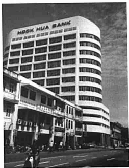
Fig. 372 Hock Hua Bank Headquarters, Sibü, officially opened in 1996. (Photo: Fong Hon Kah, 1996)
