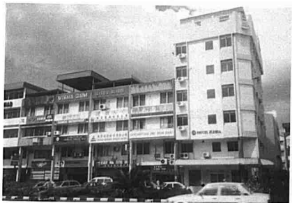
Fig. 324 The rapid development of Sibuan since the 1970's saw the former Kampung Nyabor being replaced by new concrete multi-storey shops. (Photo: Fong Hon Kah)
