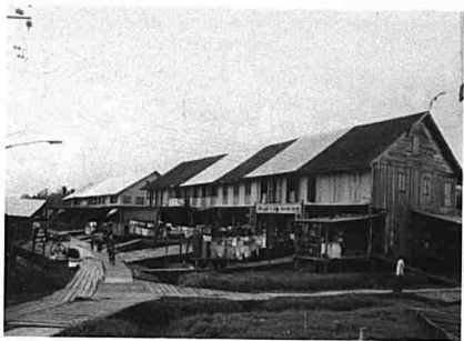
Fig. 315 Shophouses at Daro Town. (Photo: Lim Yu Seng)
