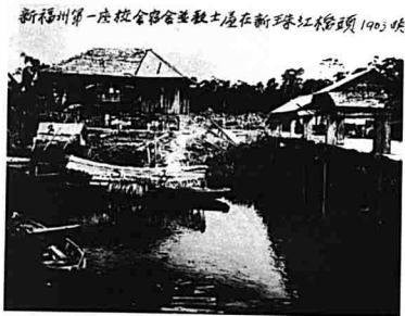
Fig. 107 The first Methodist School with dormitory for boarders and quarters for the Pastor, built at Seduan on the bank of Sungai Merah, Sibü, 1903.
