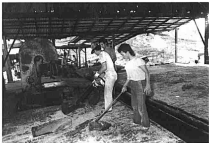
Fig. 297 Workers at the semi-mechanised sago factory, grating of sago into 'ripo' or sago saw-dust is done by machine but the extracting of sago flour is manually done. (Photo: Lim Yu Seng)
