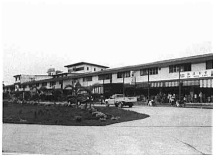
Fig. 385 New shophouses at Belaga Town. (Photo: Lim Yu Seng)
